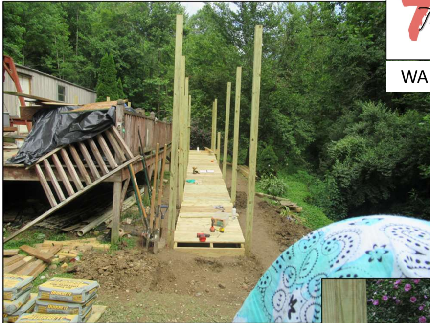
HANDICAP RAMP- IN PROCESS
